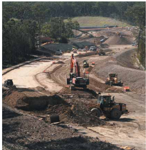
Construction works on the Cooperook to Herons Creek project.
