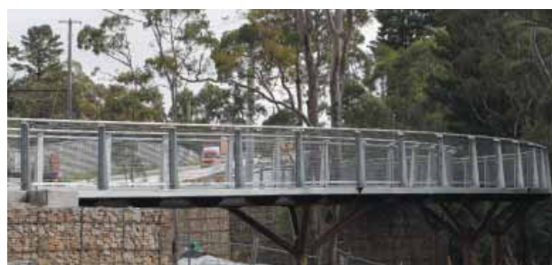
Great Western Highway at Hazelbrook. The skywalk across Gloria Park has been constructed and is opened to pedestrians and cyclists.
