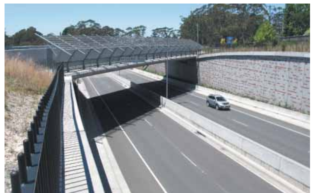
Shell Corner upgrade on the Great Western Highway, winner of the Australian Institute of Landscape Architects Design Excellence Award 2008.
