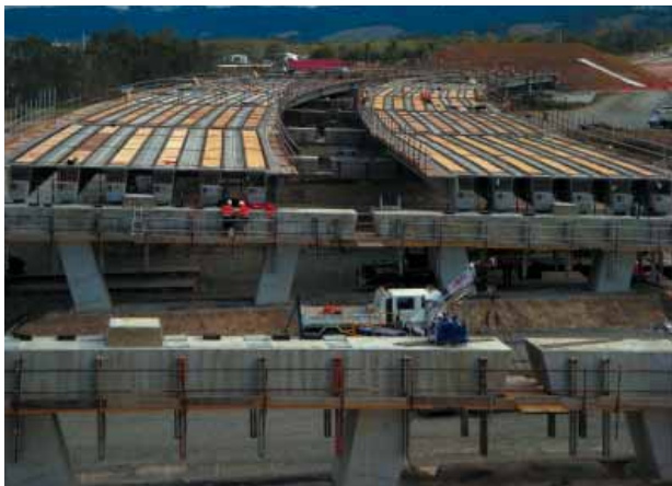
Construction works showing the placement of pre cast super-t girders on the Teven Road Bridge (360m in total length).
