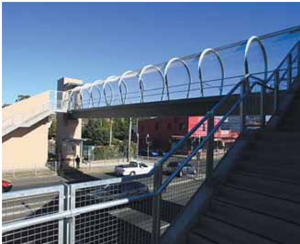
New Haberfield pedestrian bridge.
