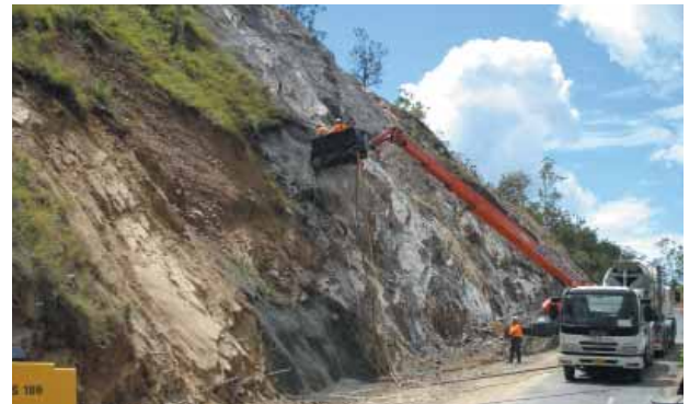
Reducing the risk of rock falls: Stabilising a section of the slope using shotcrete.
