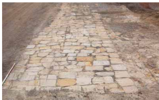
View of sandstone block road base c.1860 exposed and recorded at Leura during duplication works for the Great Western Highway in December 2008. Ref: Final Archaeological Report – Great Western Highway, Leura-Katoomba, Stages I, II and III. Archaeological Management and Consulting Group Pty Limited, March 2009.
