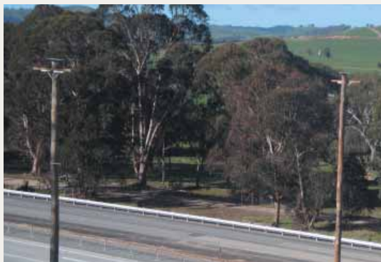
Squirrel Glider poles on the Hume Highway duplication.
