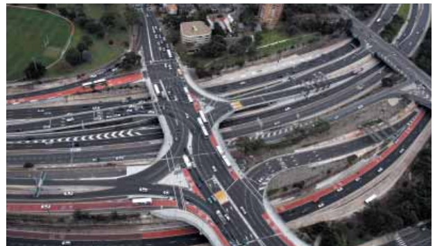
Aerial view of Warringah and Gore Hill freeways.
