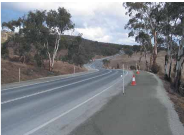
Shoulder widening along the Kings Highway.
