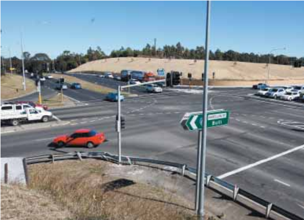
Pinch Point Program: Completion of intersection upgrade at Narellan Road, Blaxland Road and Gilchrist Drive at Campbelltown.
